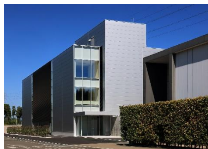
General office in Himi Plant
